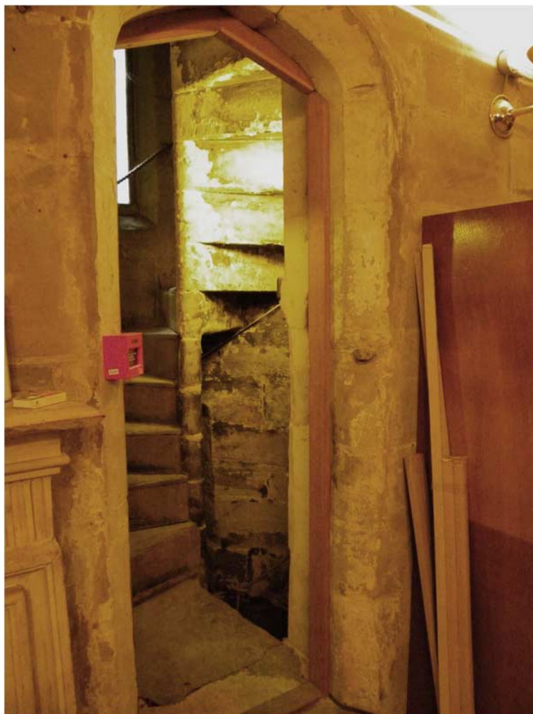
Fig 3. The vice in the north wall of the vestry. To the left is the Victorian mantle of the medieval fireplace. Photograph: author
