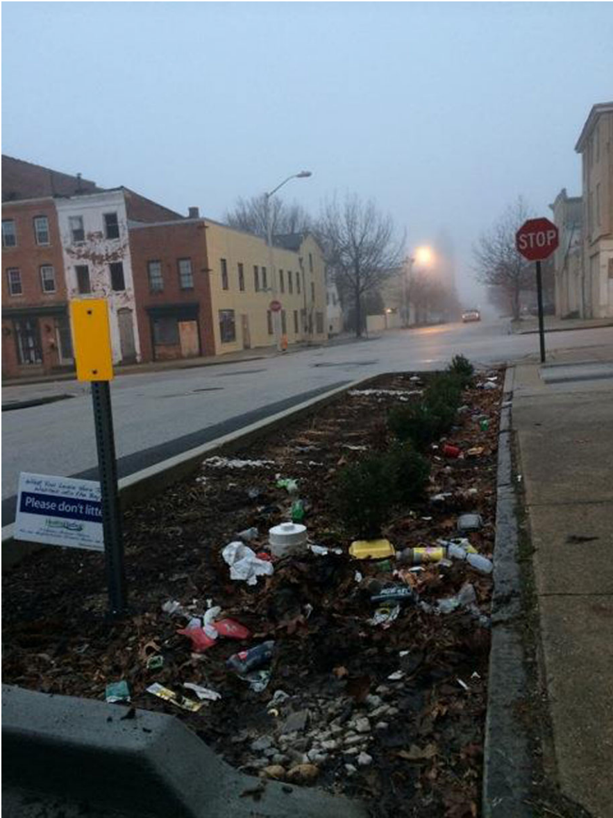
Figure 4. A green infrastructure feature in an underserved neighborhood in Baltimore, MD, USA. This feature is designed to reduce runoff to receiving waters well outside this neighborhood, which loses parking spaces. The feature has accumulated trash, despite a “please don’t litter” sign and plant material has degraded. Photo by Neil Bettez.
