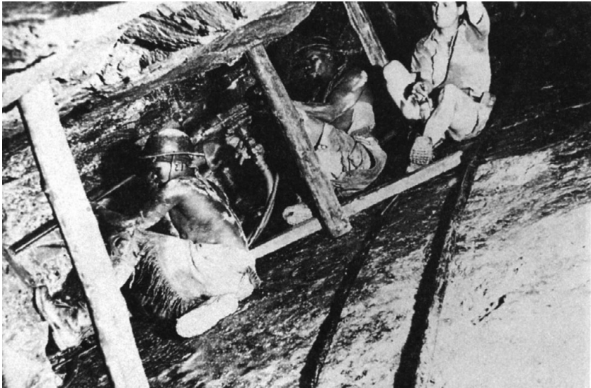
Figure 1.6 Jackhammer stoping in East Rand Proprietary Mines, 1938. Source: Barloworld Rand Mines Archive at Historical Papers Research Archive, University of the Witwatersrand, South Africa
