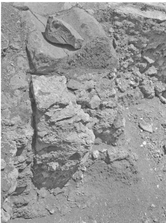
FIG. 6. View from the west of a section through the stylobate foundations of the north portico (left) and the rough foundations supporting the tuff gutter (middle) in front of the portico. To the right are deposits of rubble and debris used to create the temple terrace. (Photo: author.)
