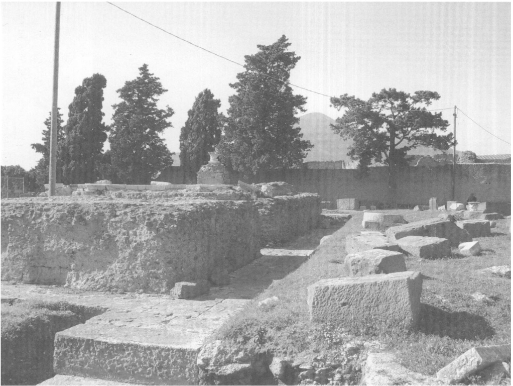
FIG. 21. View from the south of the temple as it was being enlarged after AD 62. The upright opus caementitium core is part of the mid-first-century BC temple; the still intact courses of large basalt blocks were laid into a construction trench surrounding the earliest building. The scattered basalt blocks in the courtyard are remnants of this building work. (Photo: author.)
