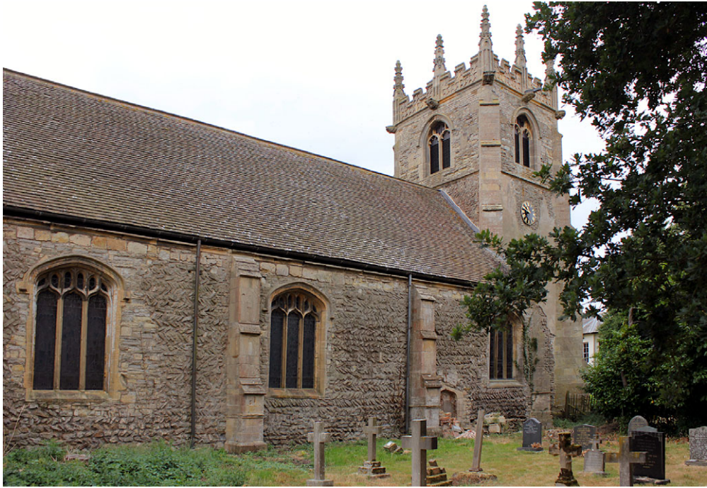
Fig 7. The church from the north-east illustrating the extensive counter-pitched rubble construction of the side walls and the small, blocked Tudor doorway in the western bay. Photograph : authors.
