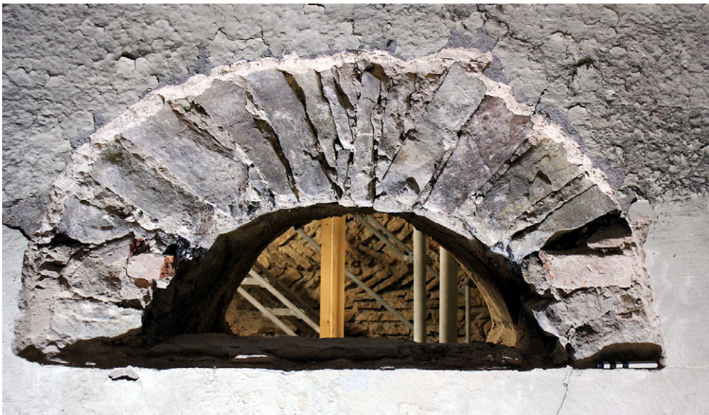
Fig 11. The east face of the blocked, rubble-headed opening. Photograph: authors.
