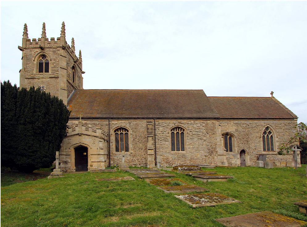
Fig 6. The church from the south showing the varied forms of rubble construction, inserted windows and the early sixteenth-century porch. Photograph: authors.
