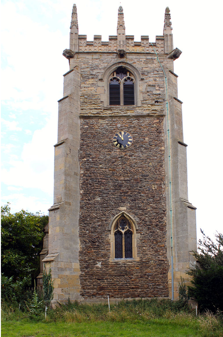
Fig 3. The west elevation of the tower showing the inserted lower window, counter-pitched rubble fabric and later medieval belfry and parapet. Photograph: authors.
