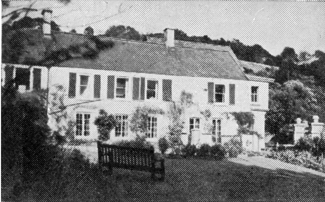
CRICKLEY COURT—ONE OF THE SEPARATE VILLAS
