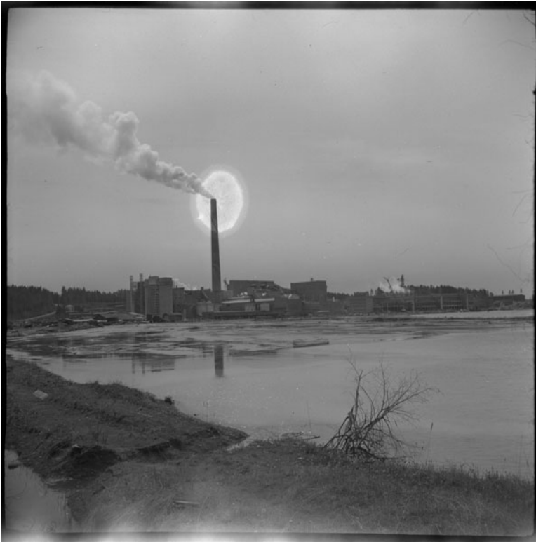
Figure 3. Kaukopää factory, 1955. The photograph depicts the timber floating area, through which logs would be floated into the plant for processing. This water was also pumped into the mill, but by the early 1970s it was fully contaminated with chemicals such as chlorine (used to bleach cellulose), leading Enso-Gutzeit to try to find a solution to pump clean river water into the plant and to send the dirty water downstream to the hydropower plant. See Erkki Vaalama, Enso-Gutzeit oy Kaukopään tehtaast, 1935–1985 (Imatra, 1985), p. 203. Photograph by Pentti Roiha. Source: Etelä-Karjalan museo, KUVKVV1499:13. Creative Commons (CC BY 4.0).
