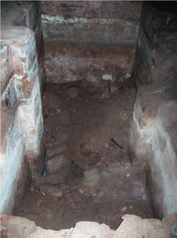
Figure 7. Cistern (photo by author, 2012).
