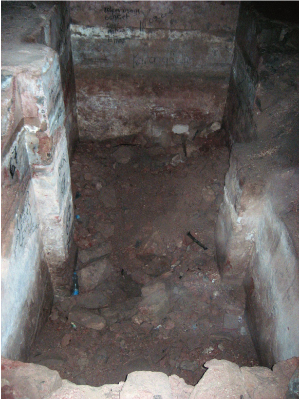
Figure 7. Cistern (photo by author, 2012).
