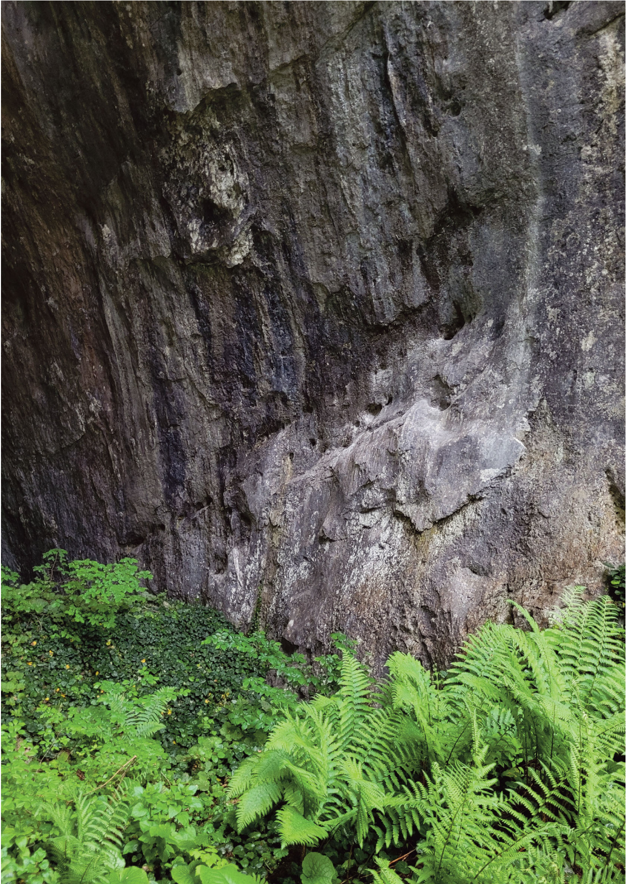
Figure 6. Remains of staircase (photo by author, 2022).
