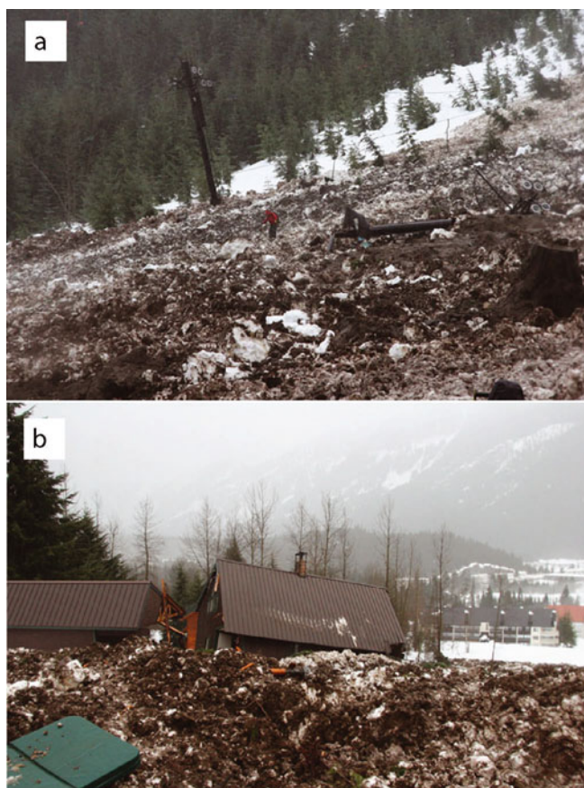
Fig. 5. Rain-on-snow event triggered an earthflow mixed with snow, Hyak Ski Area (location shown in Fig. 1b). (a) Destroyed lift tower, Hyak Ski Area. (b) Damaged houses within the avalanche run-out zone.
