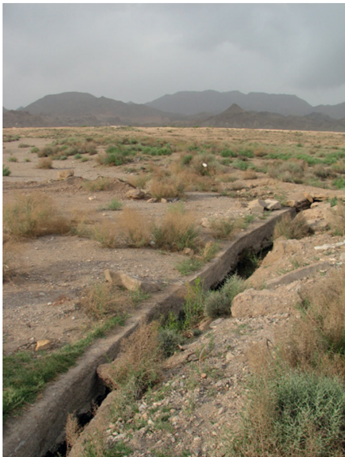
Figure 37 In Yazd, a qanat emerges to the surface after running underground for miles (photo: D.F. Ruggles)
