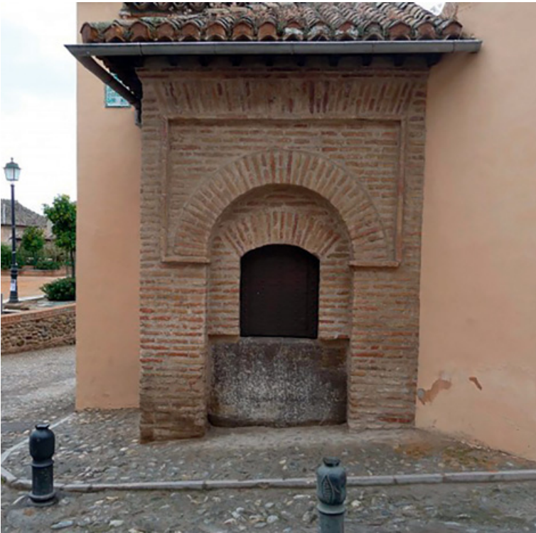
Figure 11 Exterior face of the Aljibe del Rey, Granada (photo: D.F. Ruggles)
