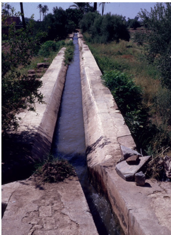
Figure 44 In the Agdal gardens outside of Marrakesh, the flow of an irrigation canal can be blocked and redirected by a simple stone barrier (photo: D.F. Ruggles)
