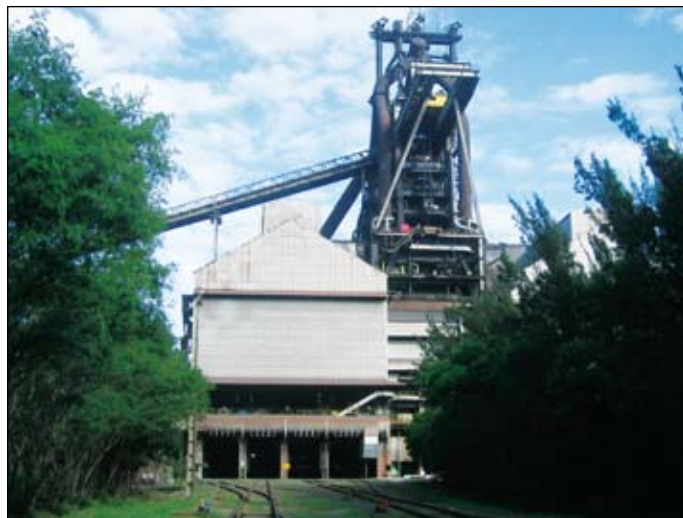
Since it came into operation in 1983, furnace 1 has produced over 85 million tons of hot metal.
