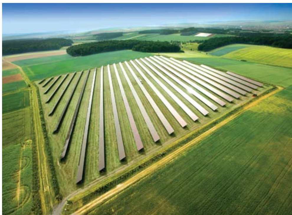
A 1.45 MW solar power plant at Dimbach in Germany, which uses CdTe thin-film cells and was constructed in 2003–2004 by Beck Energy GmbH. Courtesy of Beck Energy GmbH.
