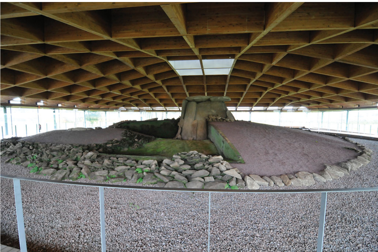
The megalithic tomb at Dombate in Galicia, Spain, within its enclosing pavillion completed in 2011 (see Editorial). The elaborate structure is designed to protect the fragile prehistoric painted decoration within the burial chamber. Photograph: Felipe Criado-Boado.
