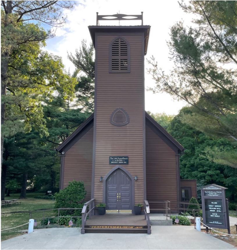
Figure 1. The Little Brown Church in the Vale. Photograph by the author.
