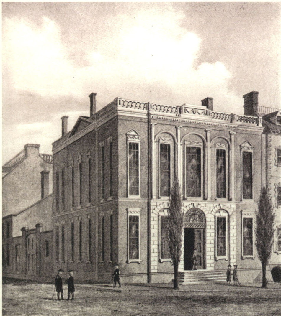
THE FIRST BANK OF NEW YORK BUILDING ON PRESENT LOCATION, 48 WALL ST.
