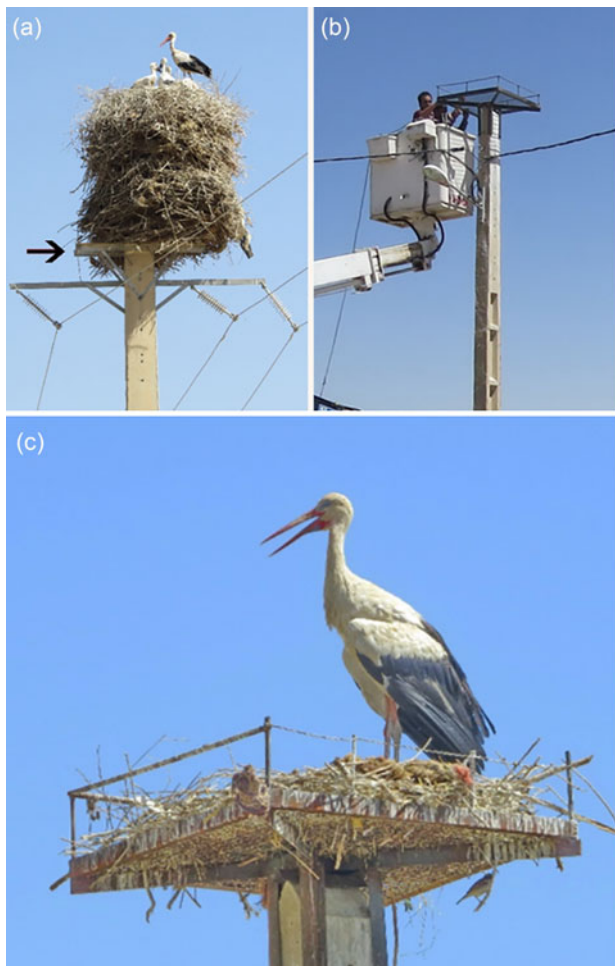
White stork Ciconia ciconia conservation project in central Iran: (a) reconfiguration of 20 kV medium-voltage power line (the arrow shows the original crossarm), (b) installation of first nest platform on 220 V low-voltage power pole, and (c) occupation of nest platform. Photos: Mahmood Kolnegari.
