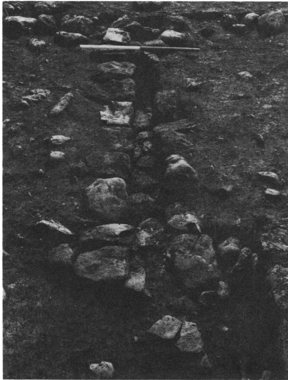
A. Culvert 1 from the north, showing deliberate blocking at the south end (p. 230).
