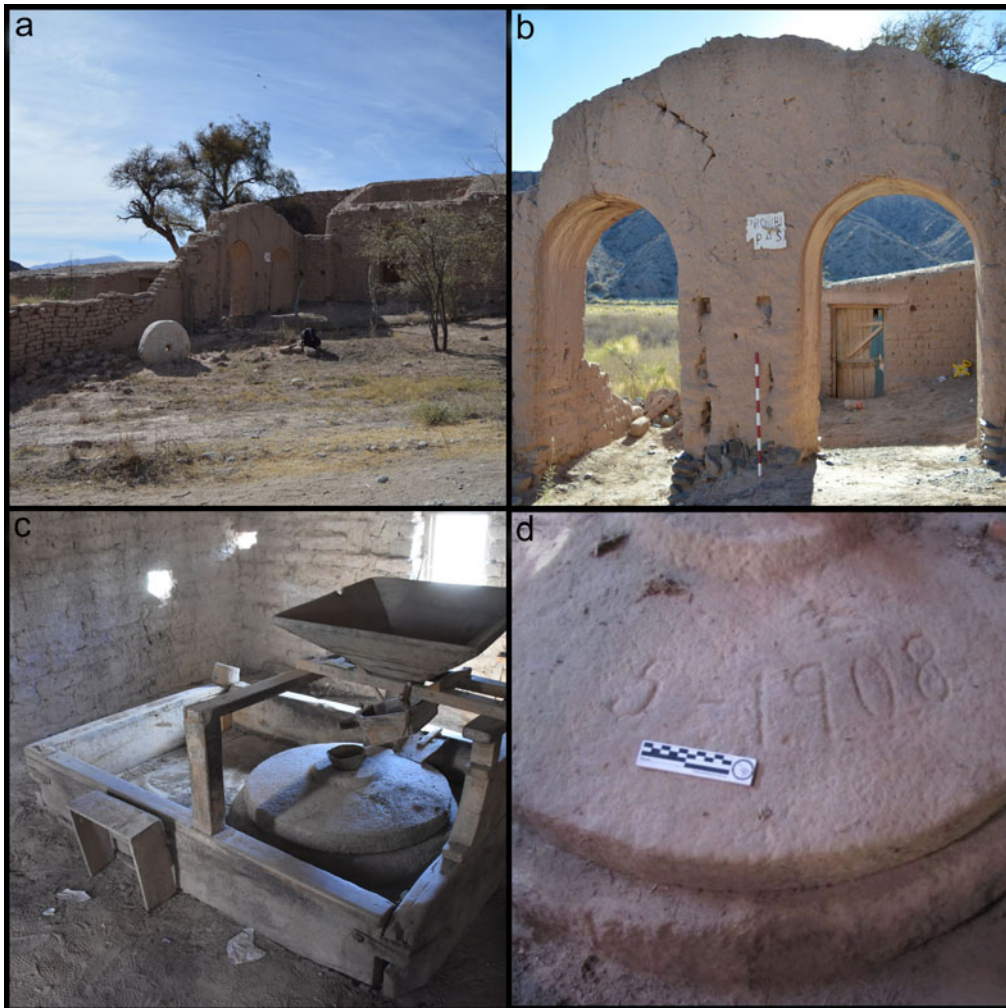
Figure 5. The Historic Mill of Payogasta: (a) the mill room and its enclosures; (b) the entrance arches (in front) and the mill room (at the bottom); (c) milling machinery; (d) detail of the flywheel of the previous figure, where the inscription of the date is engraved (photographs by Andres Jäkel and Pablo Pifano). (Color online)
