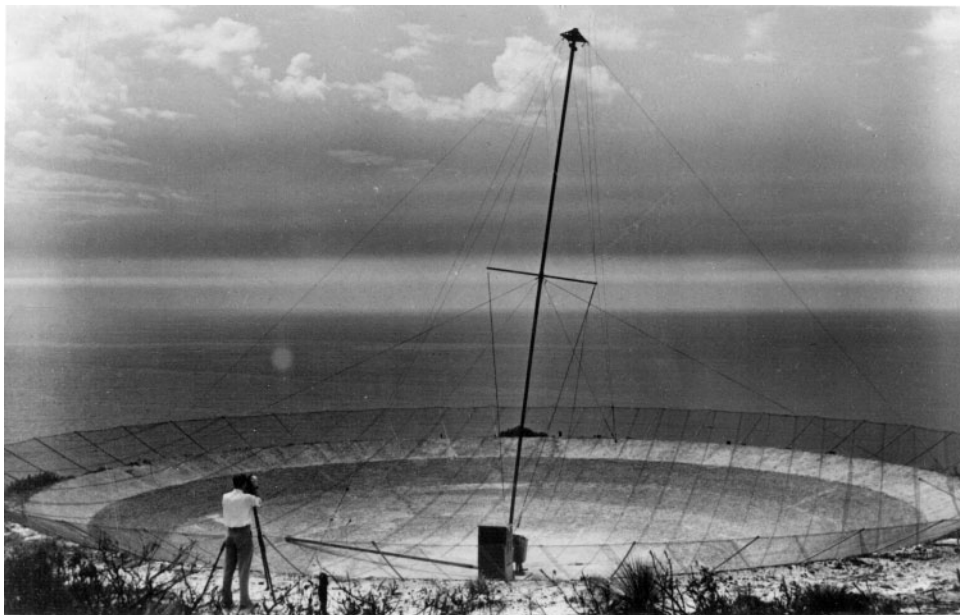
Figure 21 The enlarged concrete-surfaced 24.4-m dish during the survey in 1953, with Gordon Stanley using a theodolite to set the zenith angle of the antenna mast.
