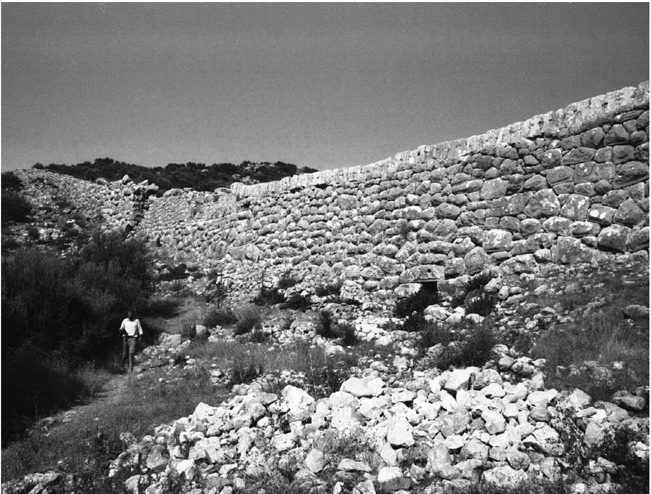
Fig. 33. Delikkemer, Patara, aqueduct above city.
