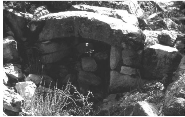
Fig. 30. Covered drain south of MI 3 looking west, in 1981 (by A.S. Hall).
