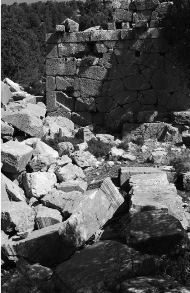
Fig. 20. YÇ 1026 and 1027 context, looking along north-western stoa towards northern corner of MI 2.
