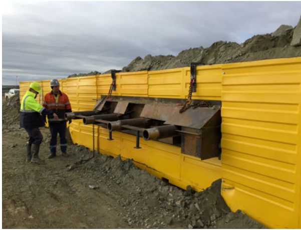
FIGURE 7. A load test frame as applied to the EP units during a physical testing at the Edna May gold mine.
