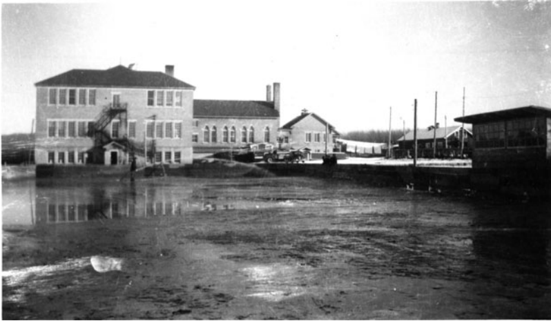
Fig. 5. Lejac Indian Residential School in the 1930s. Residential schools, built to house hundreds of Indigenous children, were often large and imposing structures. Photo courtesy of the Archives of the Diocese of Prince George, Prince George, British Columbia.
