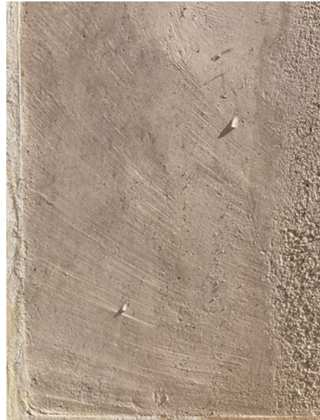
Figure 8. Polished opus signinum surface repelling water droplets. Note the trowel marks left in the process and the rougher, washed off surface, showing the difference between original finish and ‘archaeological’ state.
