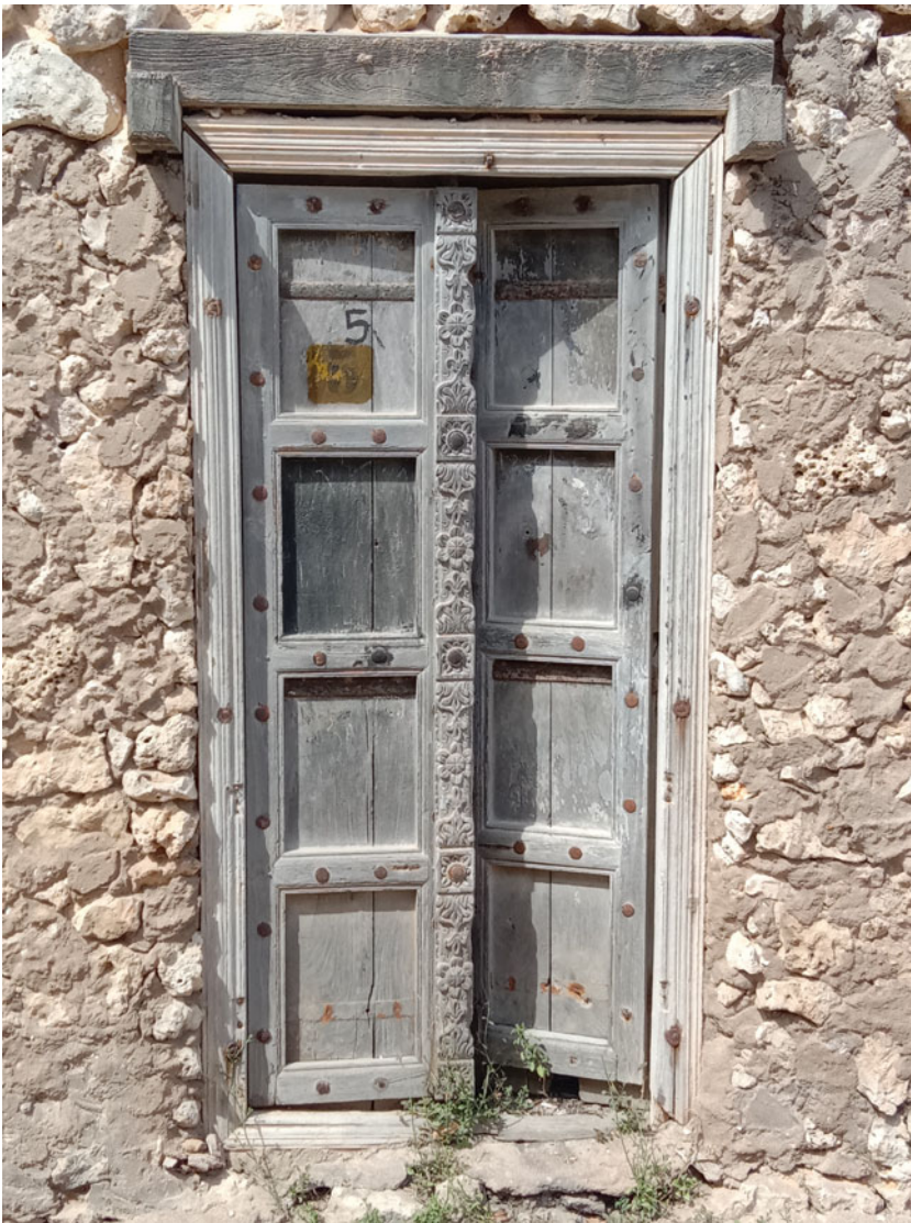
Figure 8. Wooden house door, showing the decorative use of wrought-iron nails in a Swahili Coast style, Mikindani, Tanzania, 2022. (Photo by Thomas John Biginagwa.) (Color online)
