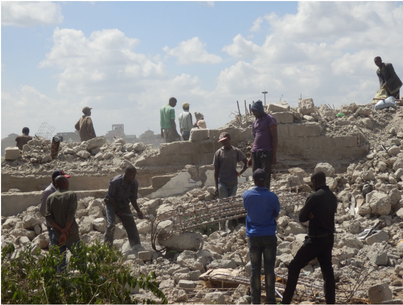
Figure 1. ‘Harvesting’ materials from a site of building collapse, for recycling and resale in Zimmerman, Nairobi, 2018.
