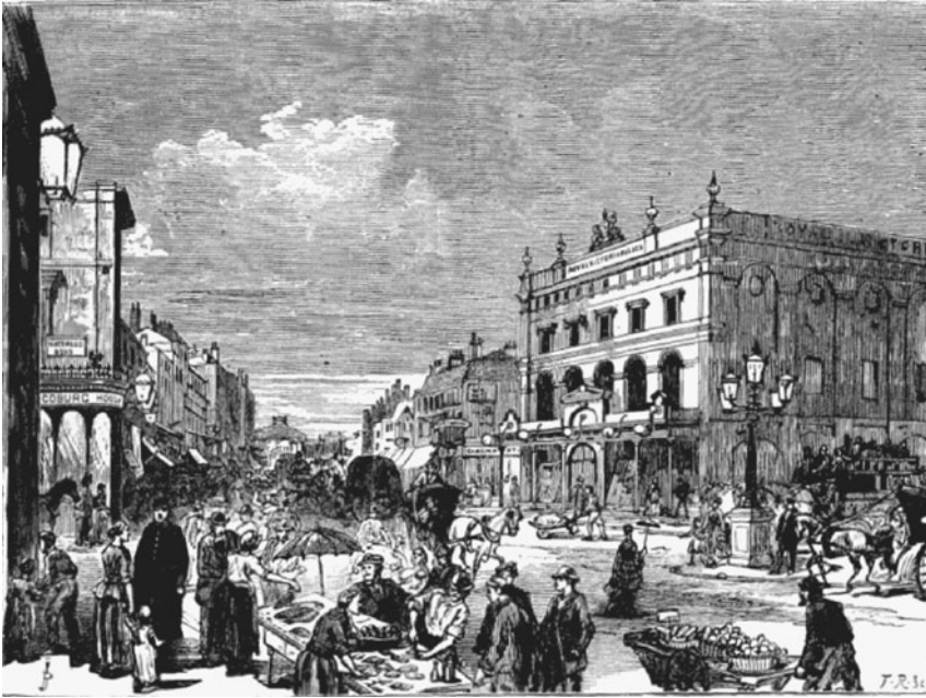
Figure 3. Though dating from ca. 1870, this scene gives a good sense of the Vic's surrounding neighborhood during Vincent's time there. © British Library Board, Wq7/8589.
