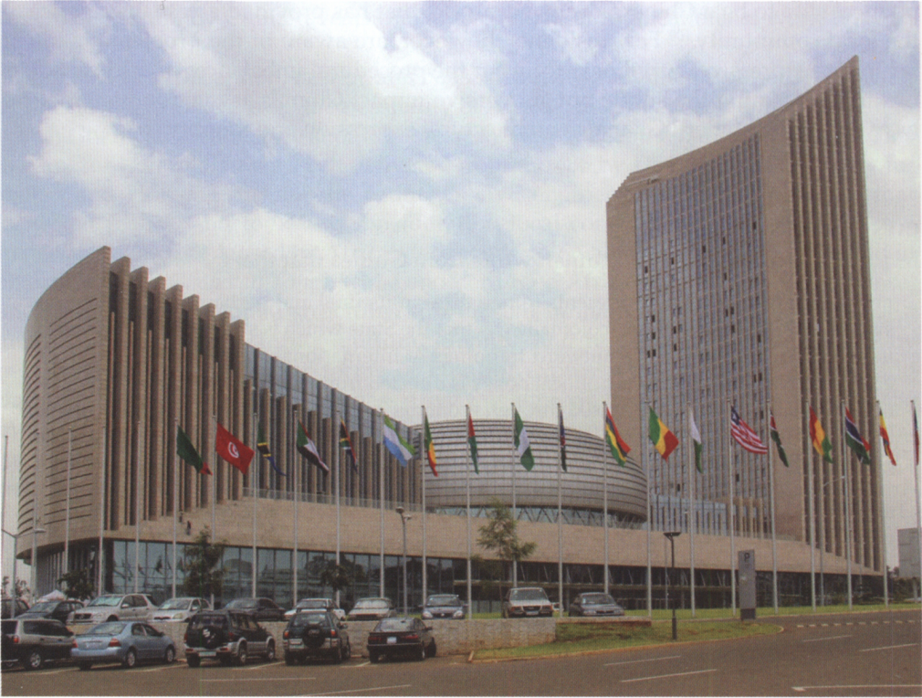
Fig. 16. African Union Headquarters, Addis Ababa (photograph of 2011; Associated Press)
