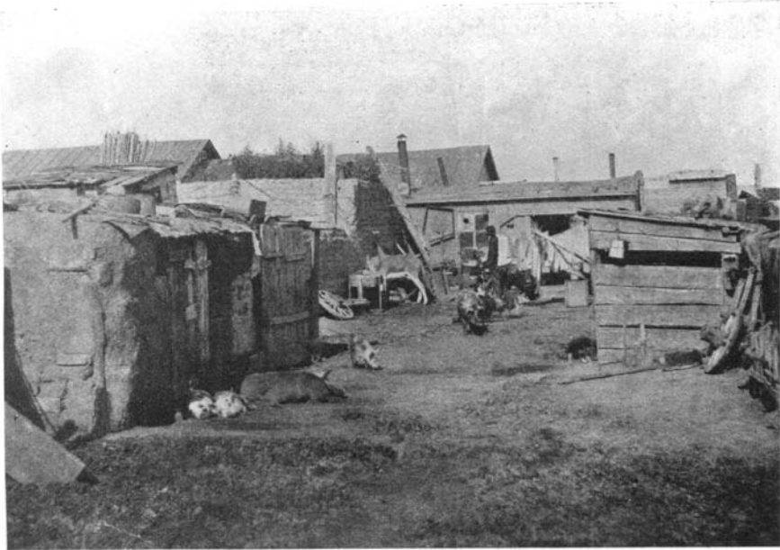
Fig. 1. Some of the inns at Manchouli. The structure seen on the right is the entrance to one of the underground type.
