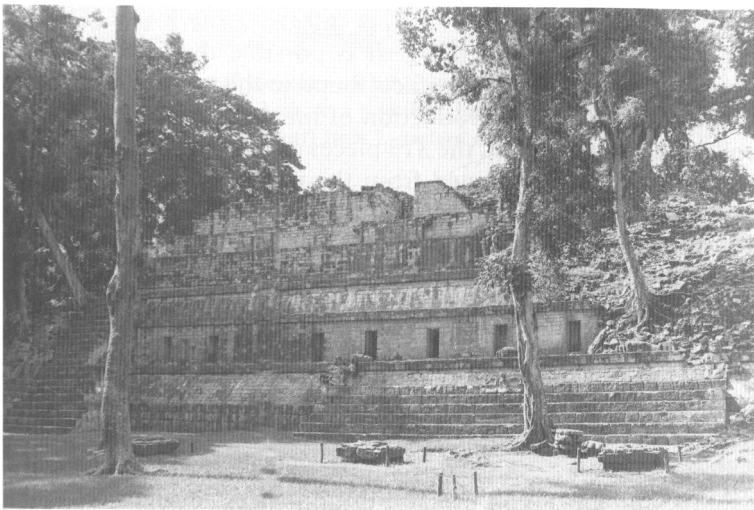
Figure 4. View of south facade of Structure 10L-11 and the West Court, Copán.
