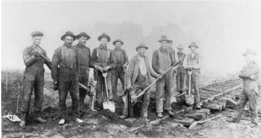
Figure 1. Finnish miners laying railway track, ca. 1910s. Industrialization created a large demand for immigrant labor in both mining and transportation.
