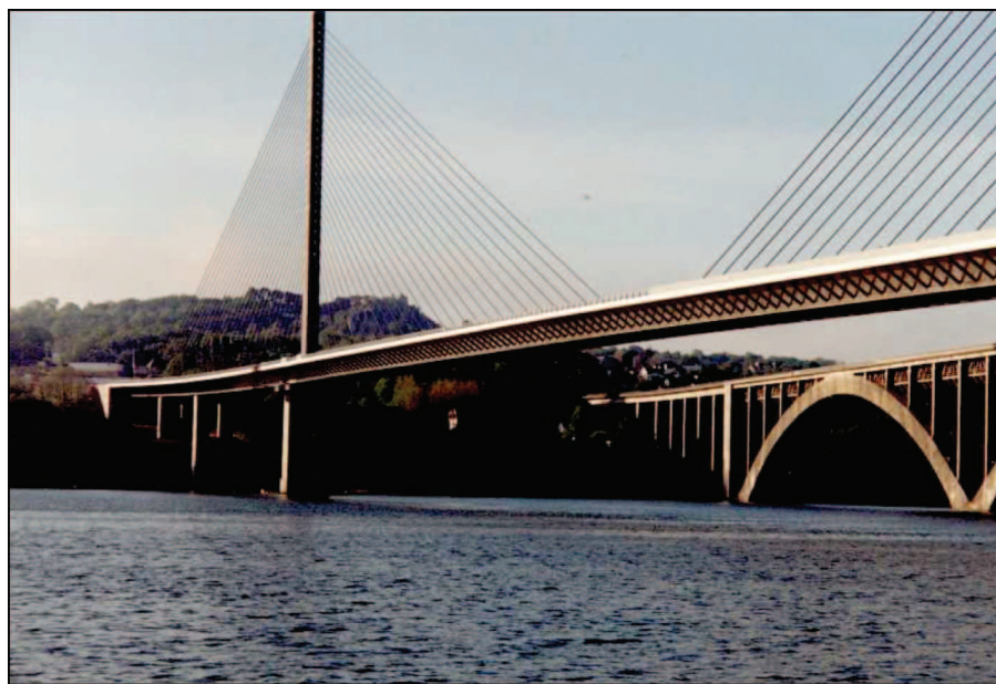
Figure 1. Two bridges built 50 years apart, spanning the Elorn River in Brittany on the west coast of France. The lighter structure of the more recent bridge (foreground) demonstrates progress in concrete construction, compared with the older bridge (background): modern concretes are ten times stronger than those of the beginning of the 20th century.
