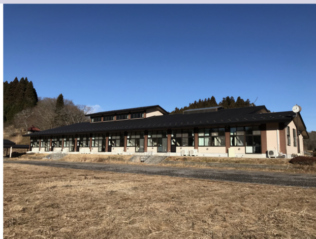
Exterior of the Long-Term Care Facility.
