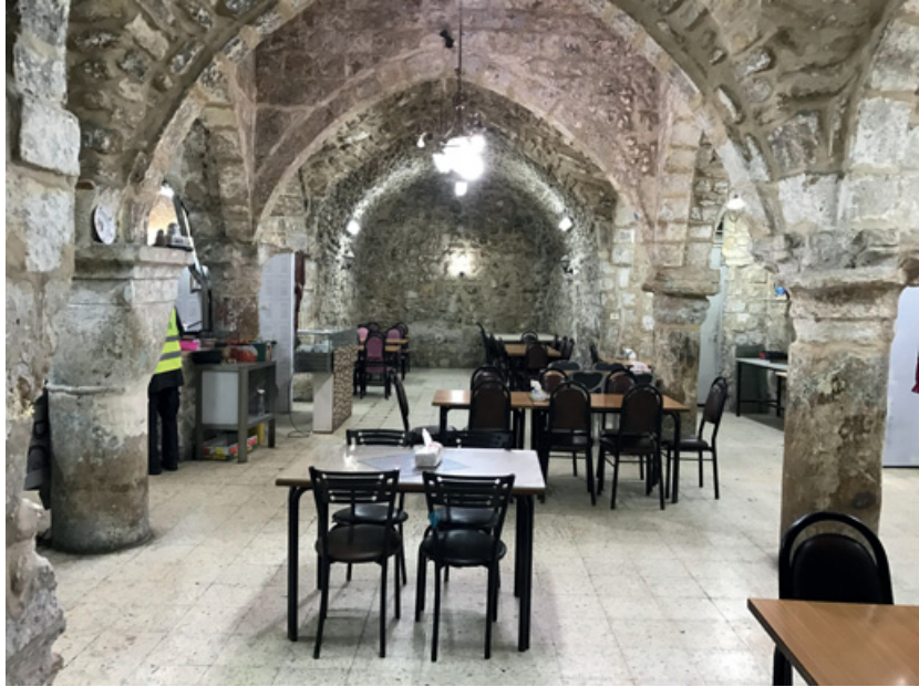
Figure 17.5 Café Bashourah: Four monolithic columns arranged in a square. Photographed by the author.
