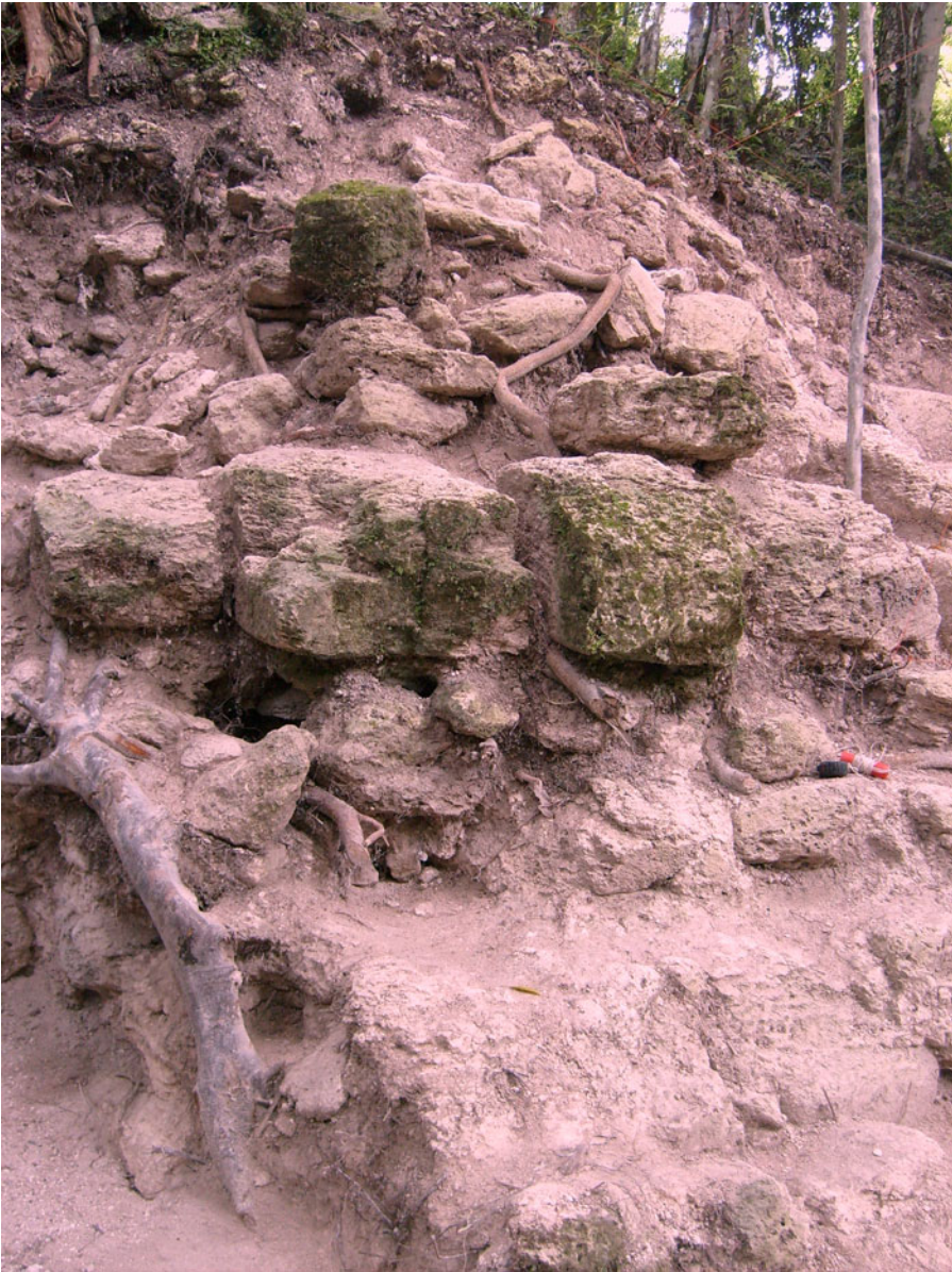
Figure 6. Destroyed mask on the east side of the fifth phase of Structure 9 (photograph by Kaitlin R. Ahern).
