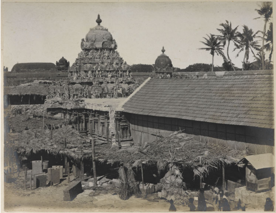
Figure 10. Main shrine to Rāmalīṅgēsvara under renovation in 1905. Source: ASI © British Library Board, Photo I008/8 (2019).
