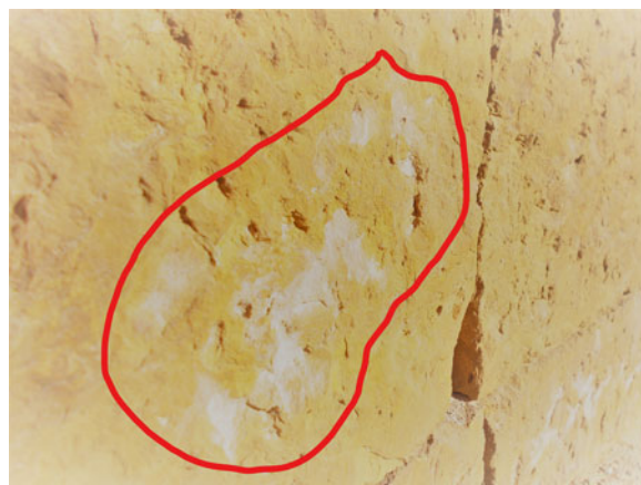
Figure 18. Efflorescence saline.
