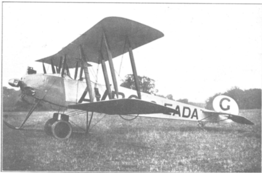
Fig. 22.—An Avro 504 fitted with an 100 h.p. Bristol Lucifer Engine.
