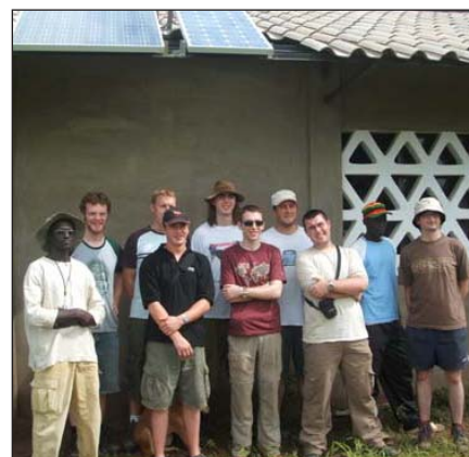
The installation team from Strathclyde University and GamSolar (front row): Ebrima Jarju, Mike Dolan, Colin Prentice, Michael Home, Malik Bah, and Matt Berrington; (back row): Ronald Mason, Peter McTaggart, Robert MacDonald, and Robert Currie.
