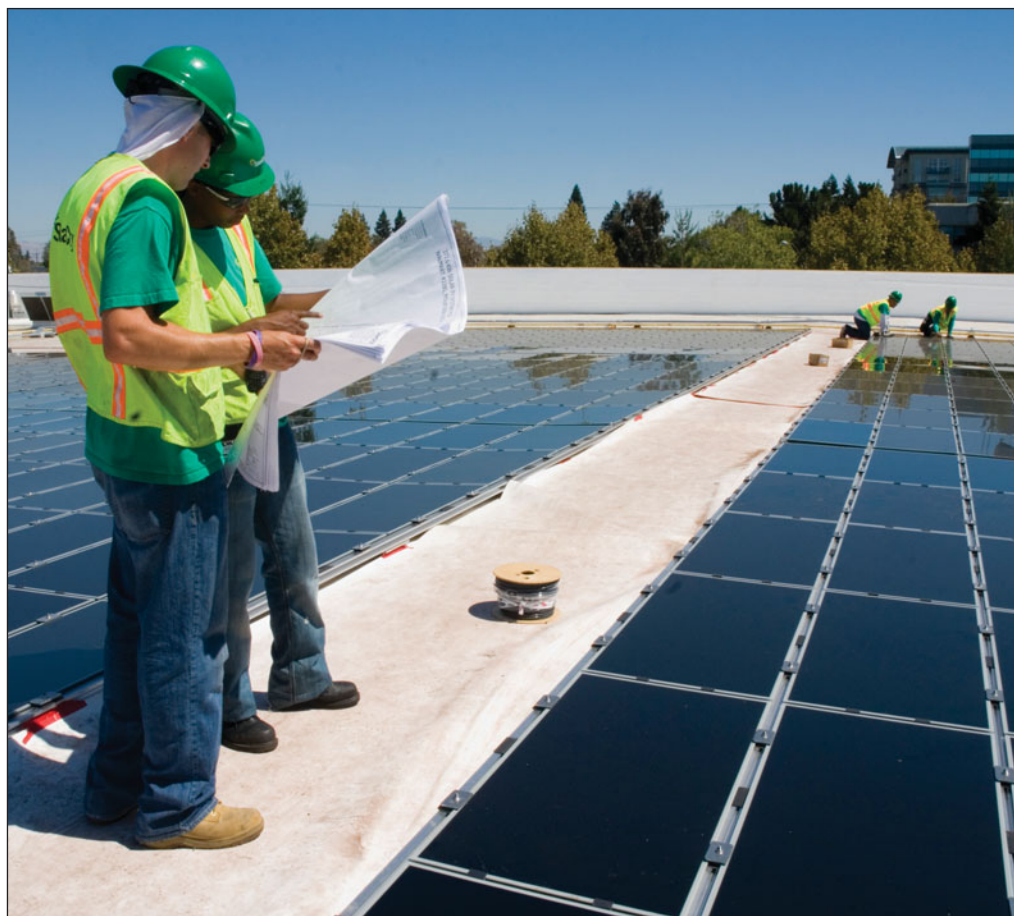
Thin-film solar panel-maker First Solar has a voluntary buyback program for its modules, which contain toxic cadmium. Something similar could be envisioned for lead-containing perovskite solar panels. Credit: Walmart Corporation.
