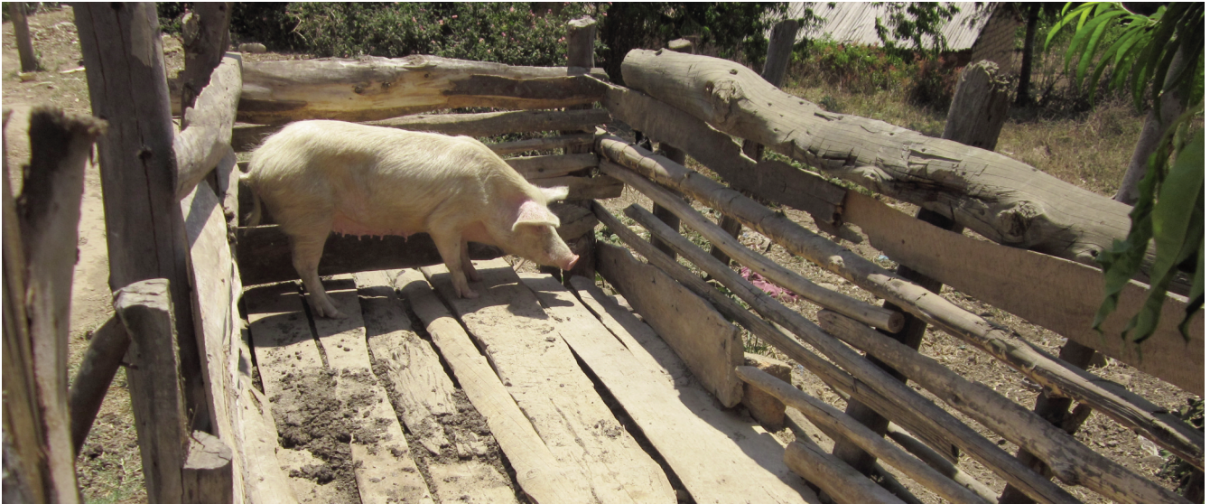
Pigs confined in a poorly constructed shelter without roof and with limited access to shade during the warmest part of the day.
