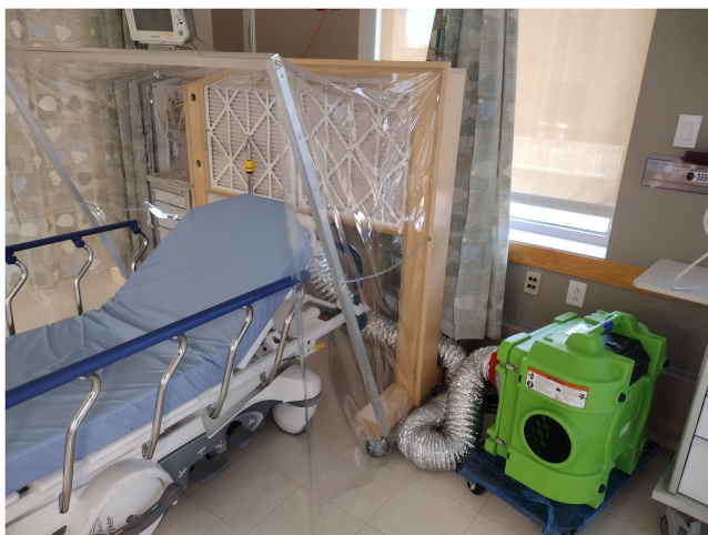
Fig. 1. Ventilated headboard device utilized at Tufts Medical Center (TMC), designed utilizing NIOSH specifications and utilized in the postanesthesia care unit (PACU).
