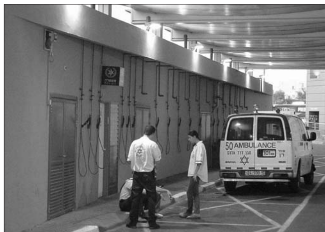
Fig. 1. Ambulance bay of a Tel Aviv emergency department. The building on the left houses security, emergency equipment, and the wet decontamination area; it also serves as a protection for the ED from bomb blasts.
