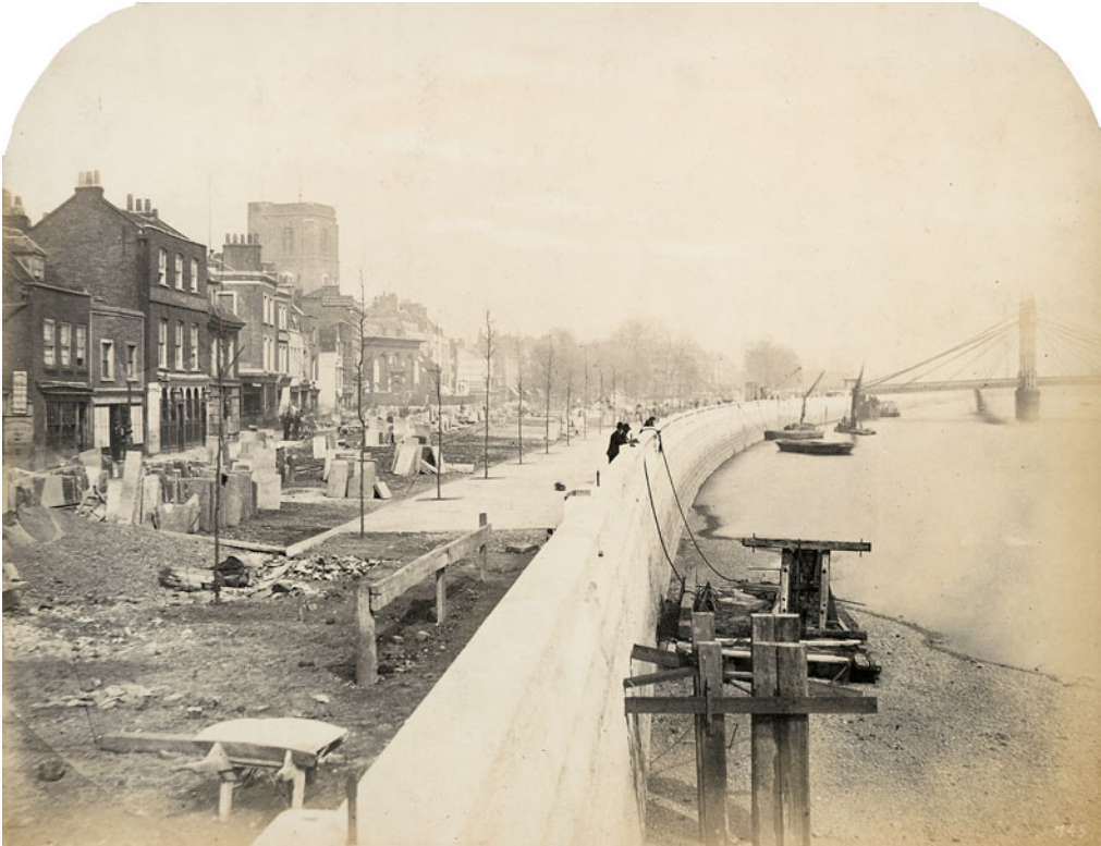
Fig. 1. Chelsea Embankment towards the Albert Bridge, 1873 (© Historic England Archive, ref: OP04624)
