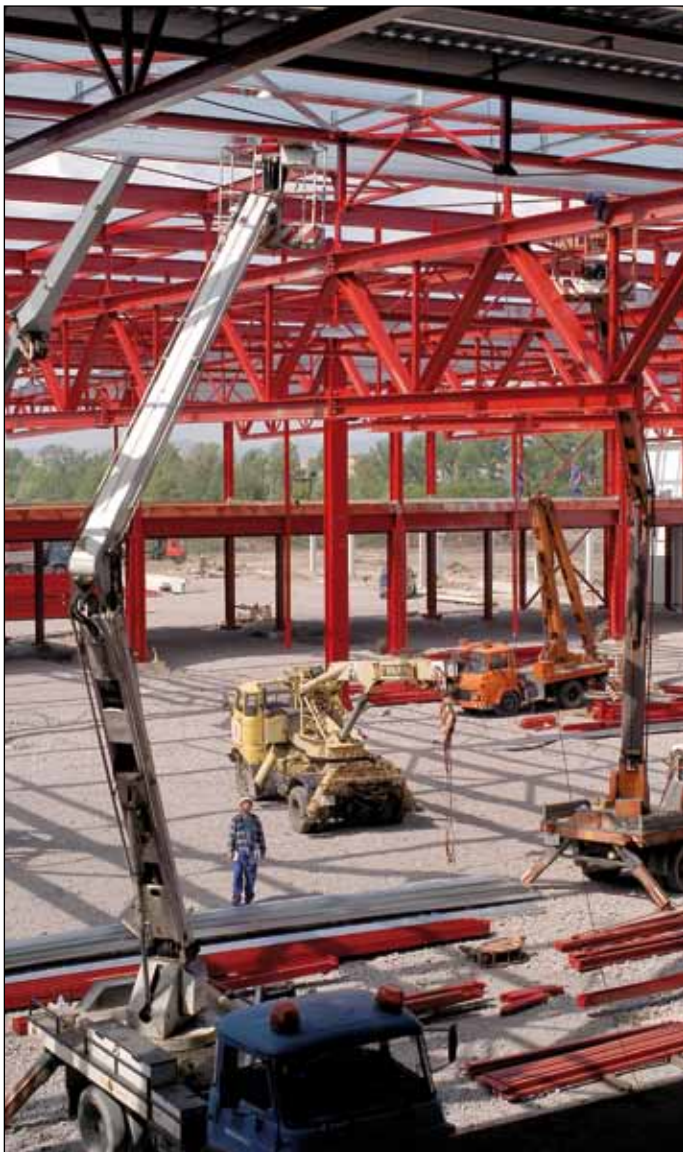
Ruukki will supply steel frame, façades and load-bearing roof structures.
