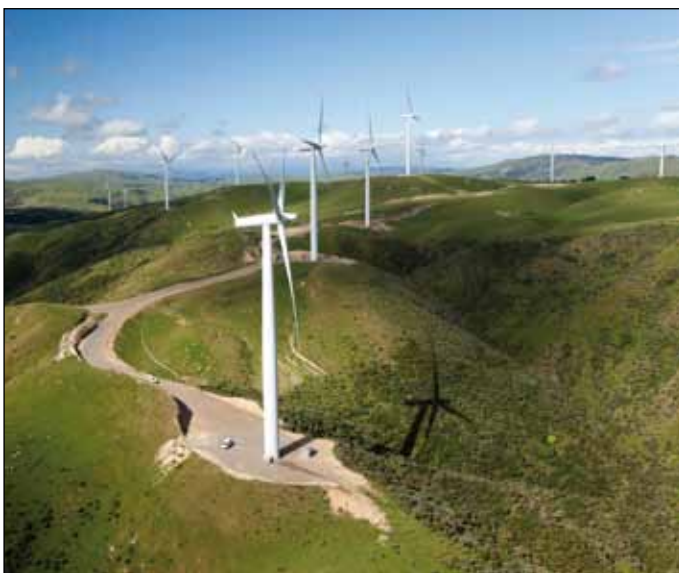
25 000 tons of profiled plate will be used to build about 150 onshore wind turbine towers. Photo courtesy of Siemens
