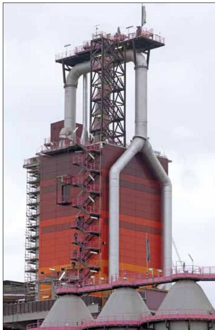
Blast furnace 9 will then be given a color cladding so as to match its twin BF8.
