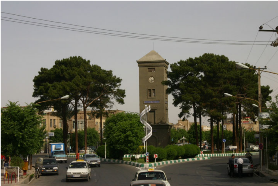
Figure 10. General view of Marker Square and Marker Clock Tower, Yazd, Iran, 1934–42. Photo: author.
