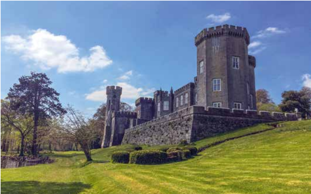
Fig. 14. Lough Cutra Castle, County Galway, Ireland, John Nash, c. 1811–17, terrace wrapping around the south and east fronts with lough visible on the left, photograph of 2015 by the author
