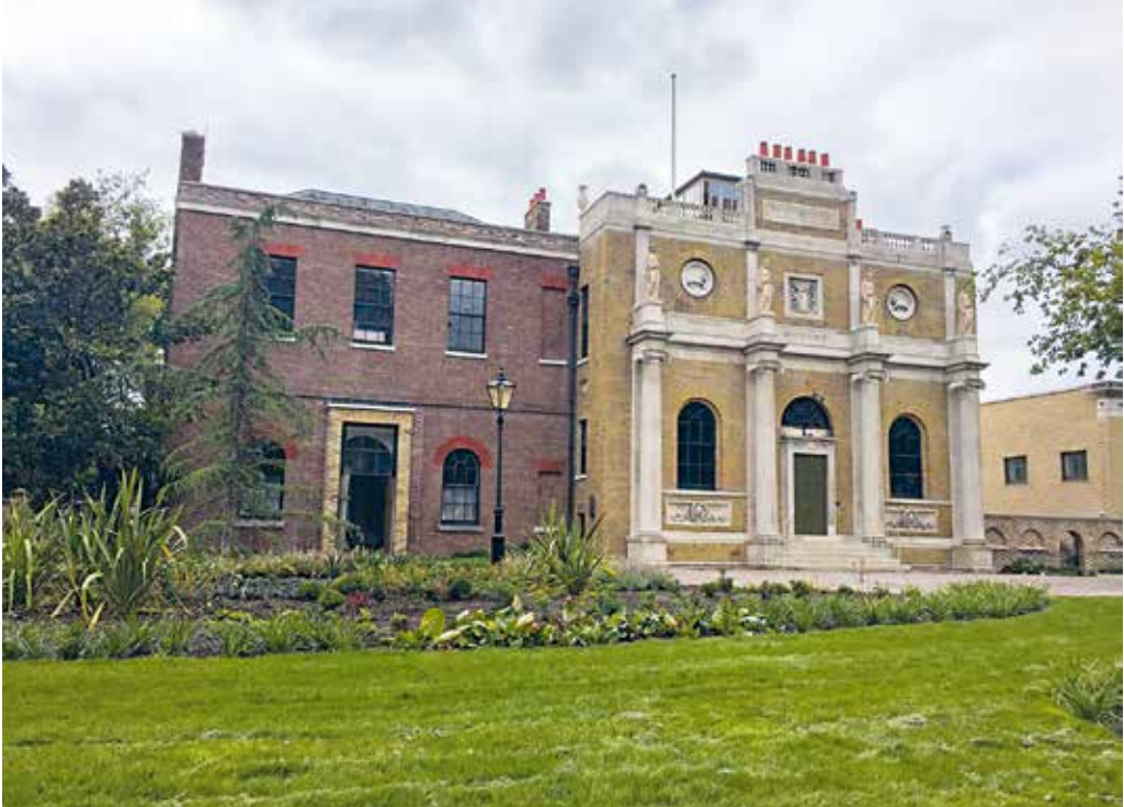
Fig. 15. Pitzhanger Manor, Ealing, London, John Soane, 1800–04, entrance (east) front, photograph of 2018 by the author
