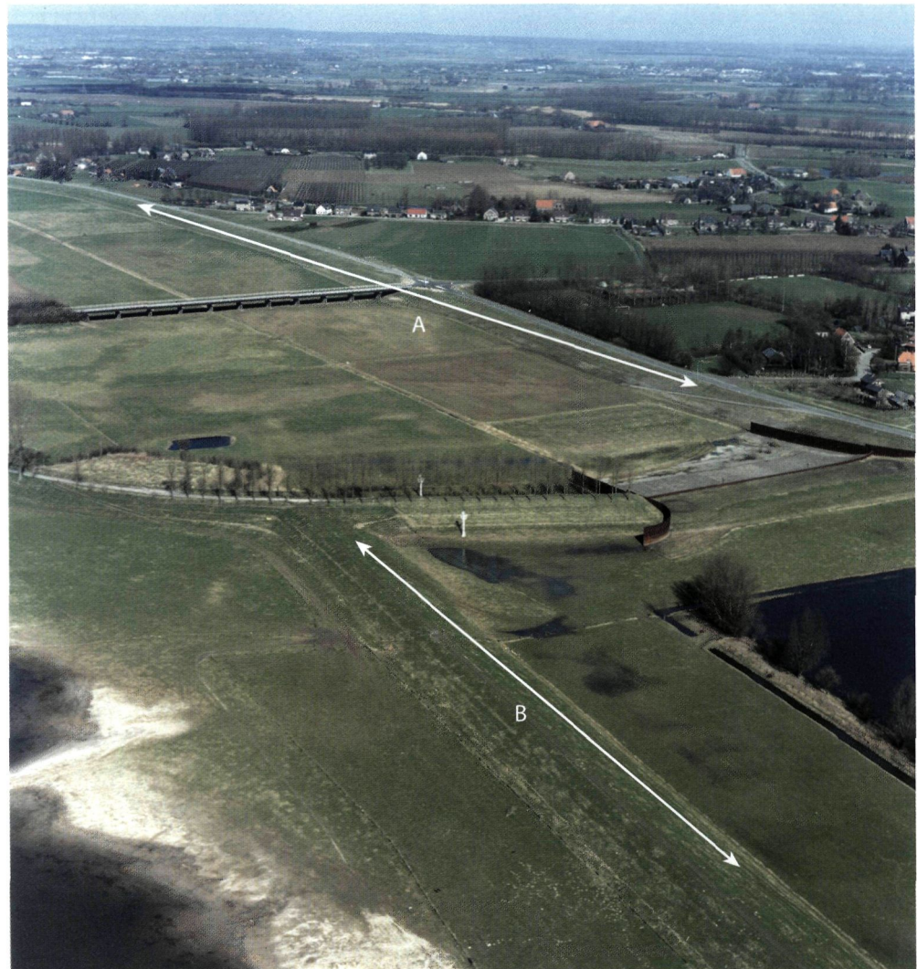
Fig. 5. The spillway at the Bovenrijn-Waal bifurcation point. The Pannerdens Kanaal flows to the left of the spillway, from bottom to top. The main dike is indicated with 'A', the summer dike with 'B'. Photo courtesy by B. Boekhoven.
