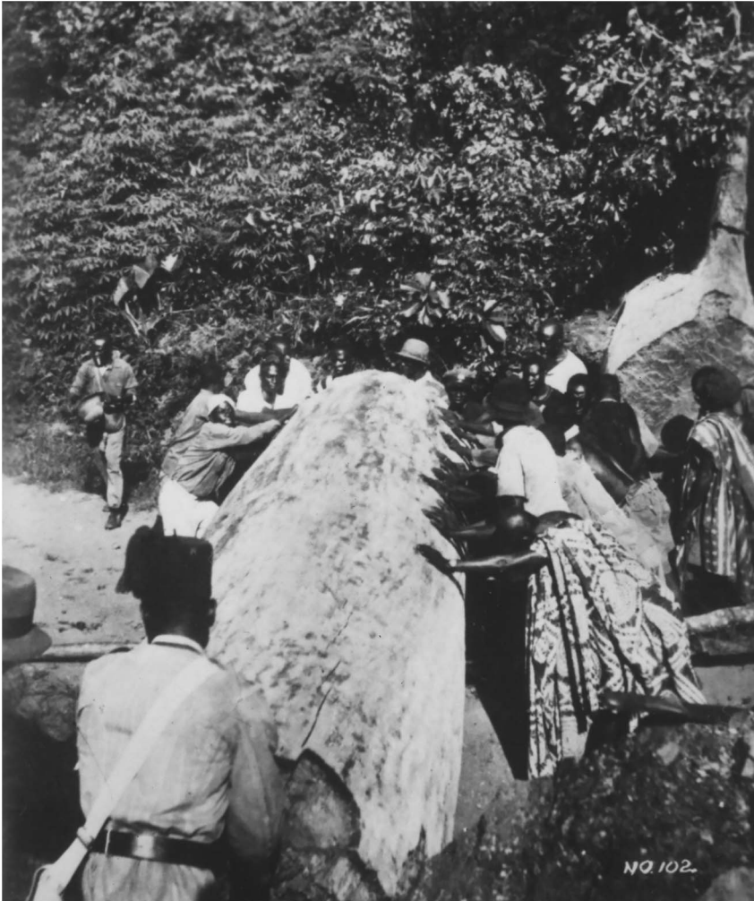
Figure 3. “Clearing a tree trunk out of the way”. Road works also included the clearance of fallen trees blocking the road.
