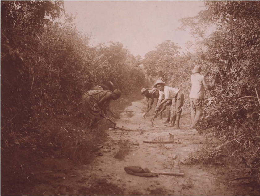
Figure 2. “Cleaning the road near Abokobi”. Road maintenance on untarred roads involved the regular weeding and trimming of trees and scrubs.
