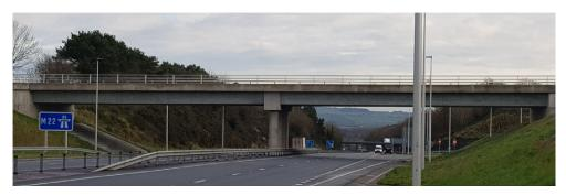
(a) A two-span beam-and-slab bridge example from Northern Ireland.
