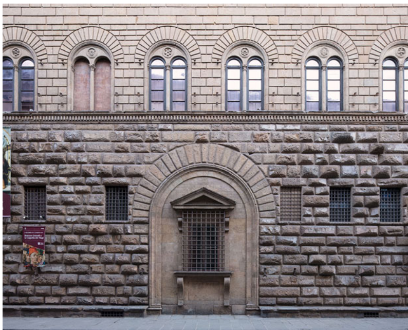
Figure 5. Palazzo Medici, Florence. Detail of facade, showing rough rustication of the ground floor. © Flavia Rossi.
