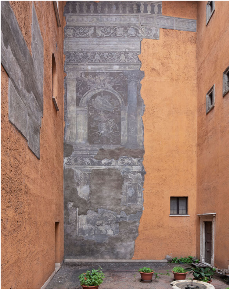
Figure 4. Palazzo dei Penitenzieri, Rome. Detail of facade, showing fragment of original incised stucco. © Flavia Rossi.
