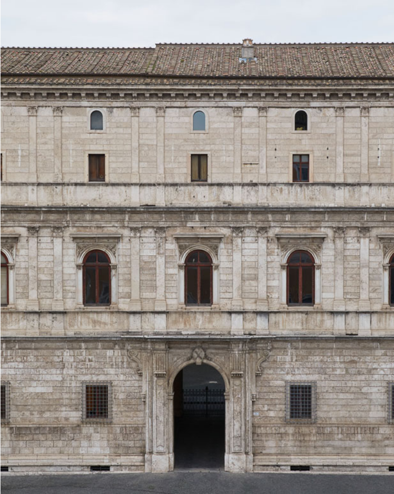
Figure 3. Palazzo Giraud-Torlonia, Rome. Facade in travertine. © Flavia Rossi.
